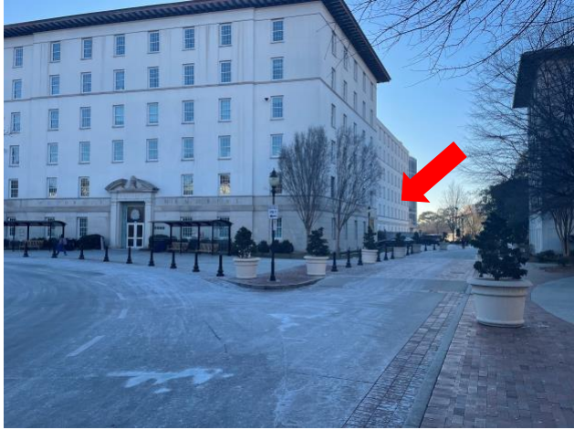
Figure 5: front doors of WMB Building
