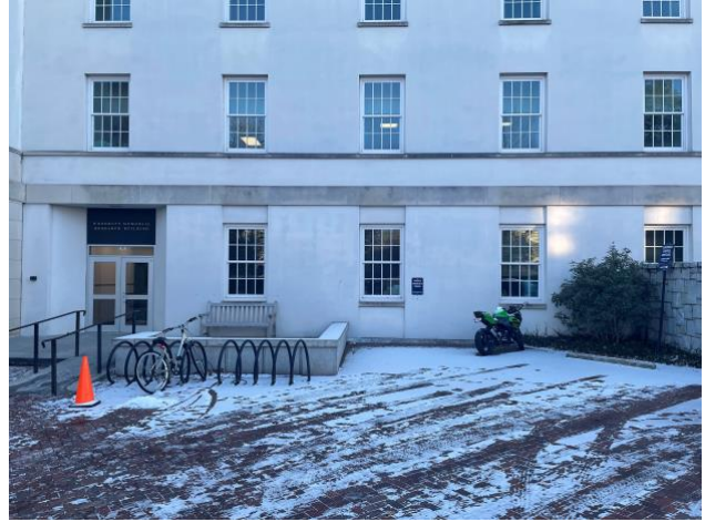
WMB Side Entrance for Deliveries (red arrow)
